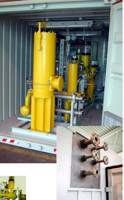
Valve Station for Gas Turbine with multicyclon separator, heat exchanger, filters and safety shut-off device
